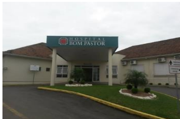
Figura 22 – Fachada Hospital Bom Pastor
