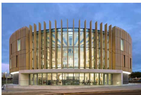
Figura 63: Fachada Principal – Rio Tayne
