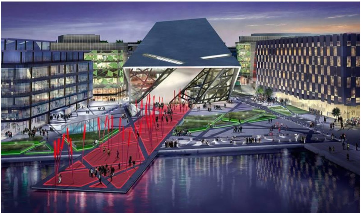
Figura 106 - Grand Canal Square Theatre and Commercial Development - Daniel Liebskind (Fonte: STUDIO DANIEL LIEBSKIND, 2010)
