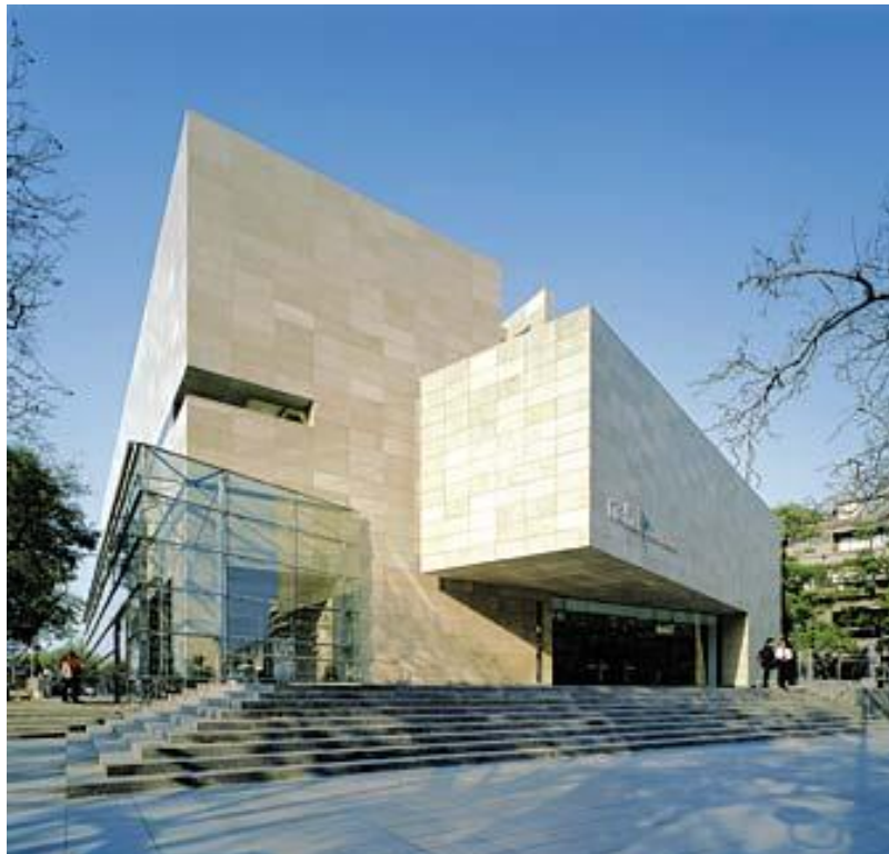
Figura 8.2.1. – Fachada Principal (ARCOWEB, 2010)
