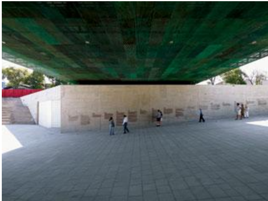
Figura 8.3. – Vão sob o volume principal (ARCOWEB, 2010)
