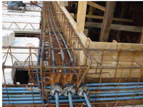
Figura 8.10: Laje Protendida (CONCREFATO, 2006)
