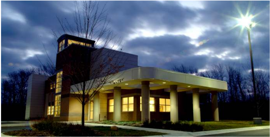
Figura 98 Hospital Veterinário North Central Veterinary Center
