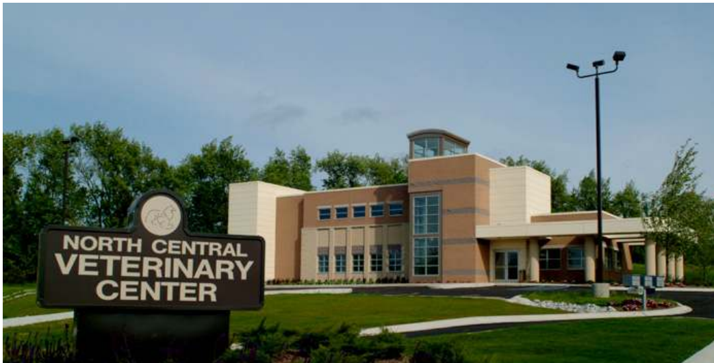
Figura 97 Hospital Veterinário North Central Veterinary Center
