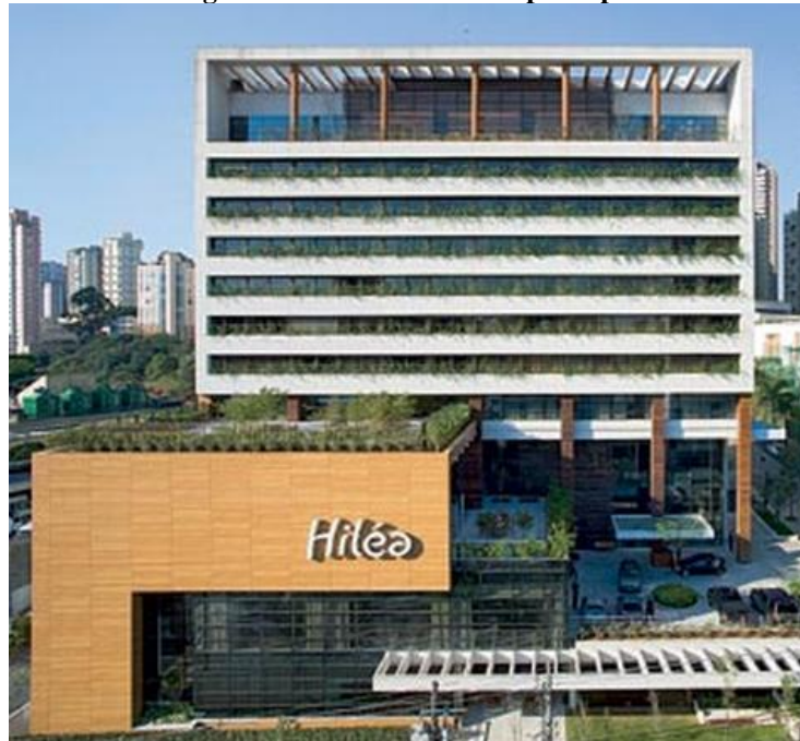
Figura 71 - Hiléa - Fachada principal
